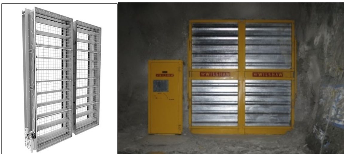
Figure 16-44 Example of Ventilation Louvres care of Clemcorp and Wilshaw
