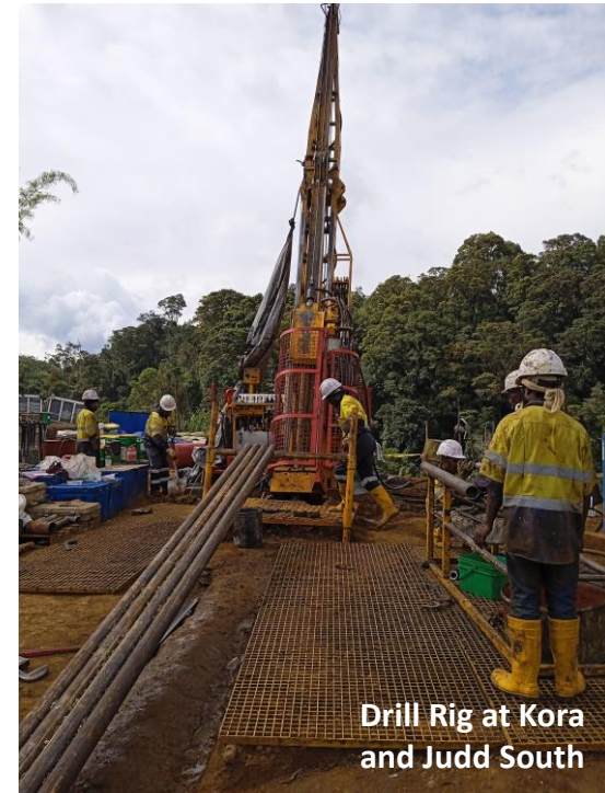
New Equipment Operating in Twin Incline
